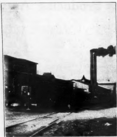
Railroad Approach to Plant
